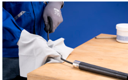
Degrease the core with a non-linting cleaning cloth.
